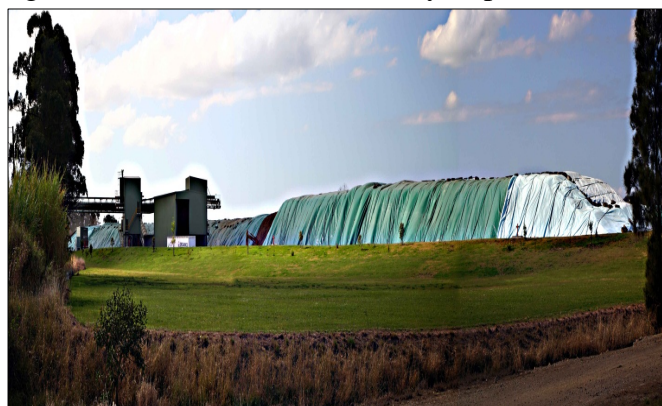
Bagasse and other biomass stockpiled at Condong Mill (NSW Sugar) for cogeneration purposes. The low bulk density makes the size of these stockpiles
