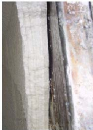
Figure 2. Build up of fouling on a vessel wall
