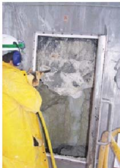
Figure 3. Removal of deposit from a scrubber
